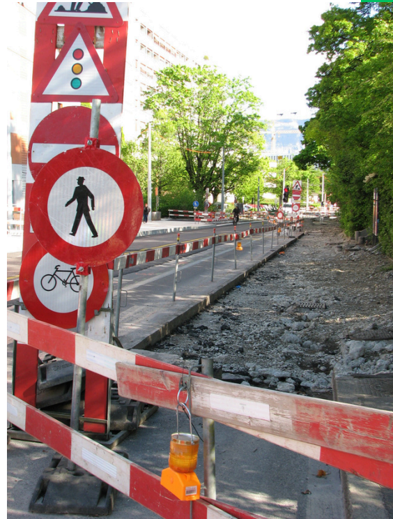
Route des Franchises, orientation sud
